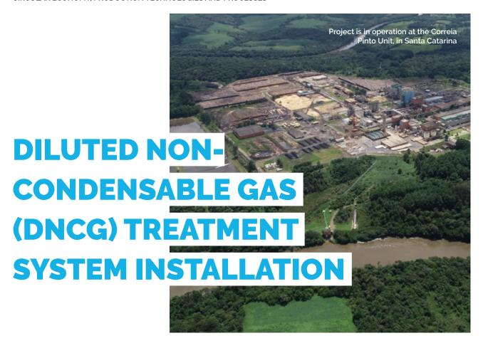
Klabin deployed a collection, transportation and incineration system for diluted non-condensable gases (DNCG) from several sources in previously mapped areas, corresponding to the evaporation, caustification (lime kilns) and pulp processes at the Correia Pinto Unit (SC). The project, carried out from July 2018 to July 2019, as geared towards reducing the odor of gases from production and benefit the communities surrounding the plant.
